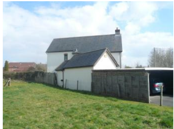
View looking north towards Coppice House
