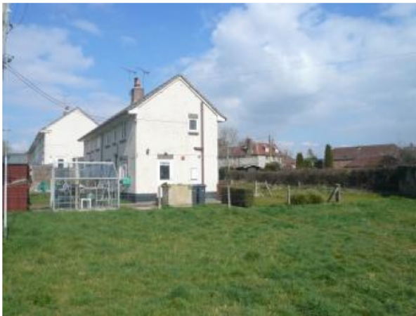
View looking north towards Park Houses and the site entrance
